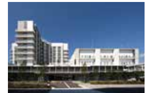
Kobe City Medical Center General Hospital
